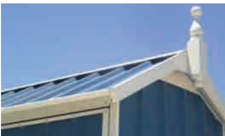
CLOSE UP OF FINIAL AND BARGES
